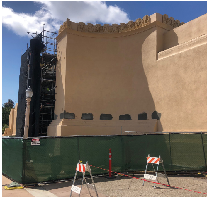
Scaffolding and application of ornamentation in progress. Photo Roger Showley.
