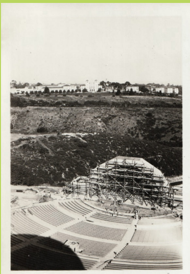
Ford Bowl under construction 1935. Photo contributed by C100 member Jim Milch.
