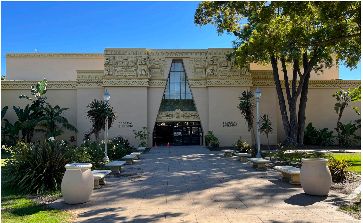
The federal Building/Comic-Con Museum fully repainted in the original colors, "Bagel" and "Honeymoon." Photo C100.
