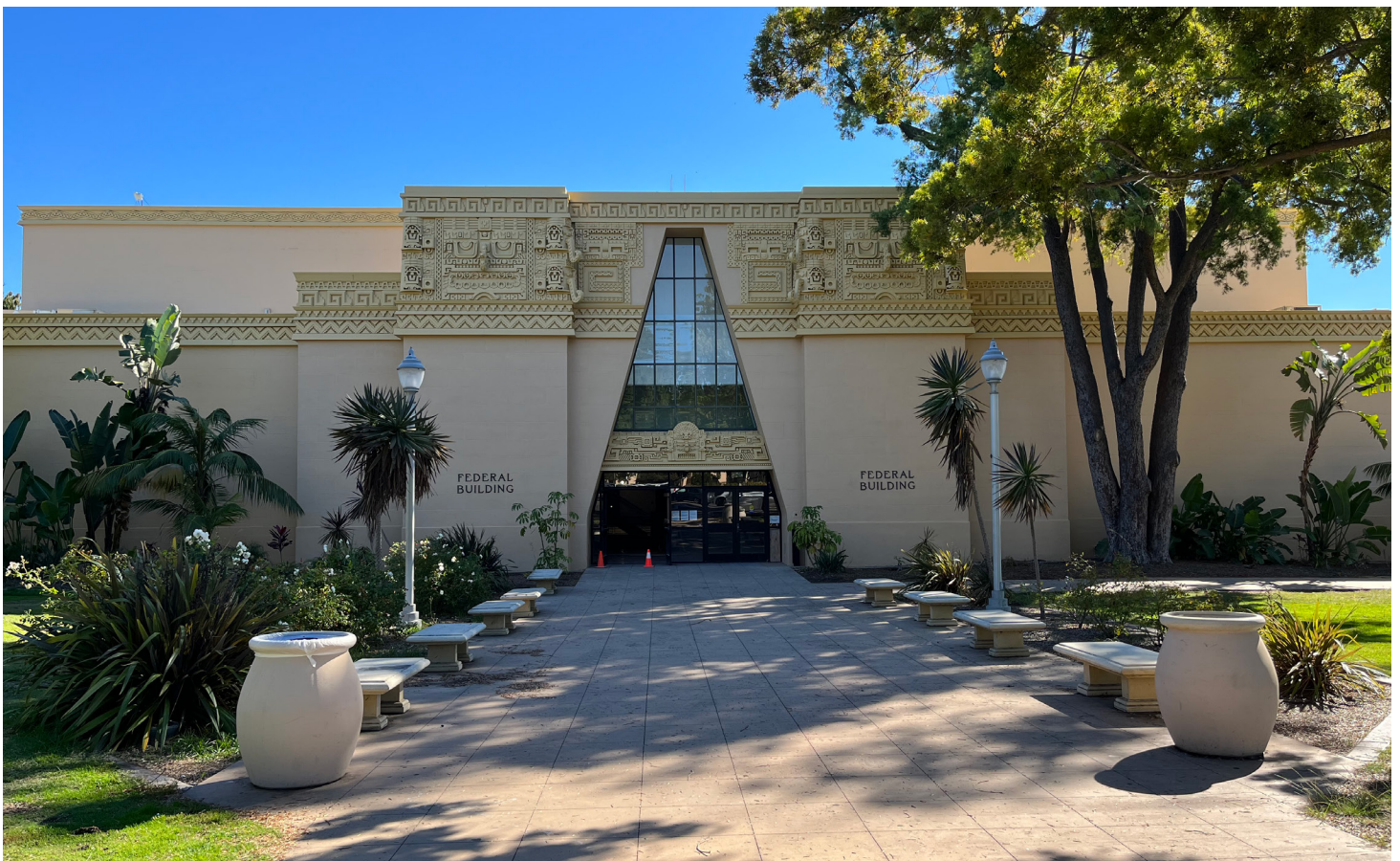
The Federal Building/Comic-Con Museum fully repainted in the original colors, "Bagel" and "Honeymoon." Photo C100.
