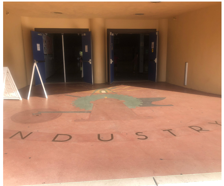
The entrance to the Municipal Gym/Palace of Electricity and Varied Industries (1935) includes this terrazzo-like treatment that will be restored in 2022 along with other artistic elements. Photo C100.
